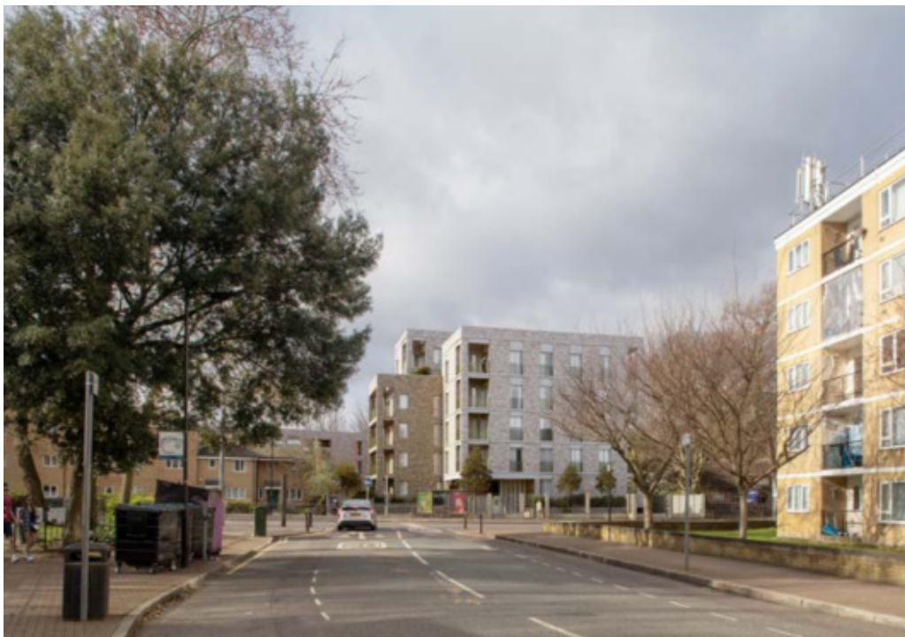
View of Block A from Neptune Street
