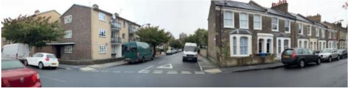
Image: View 5 showing the existing view and proposed view (The visible aspects of the buildings are outlined in a dotted blue line, and the aspects not visible are the non-dotted blue line)
